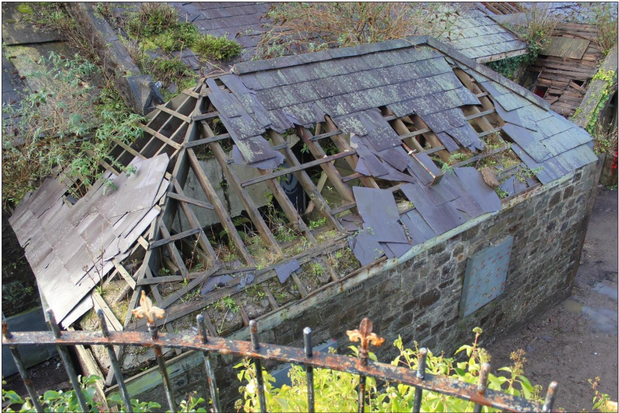
Plate 13: Hip-roofed sacristy extension to east side of northern elevation
