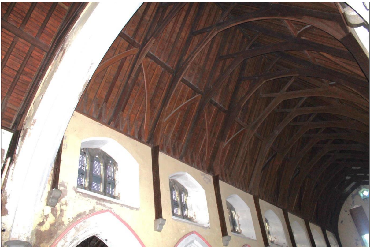
Plate 26: Detail of scissor-truss roof and southern clearstorey from beneath chancel arch.
