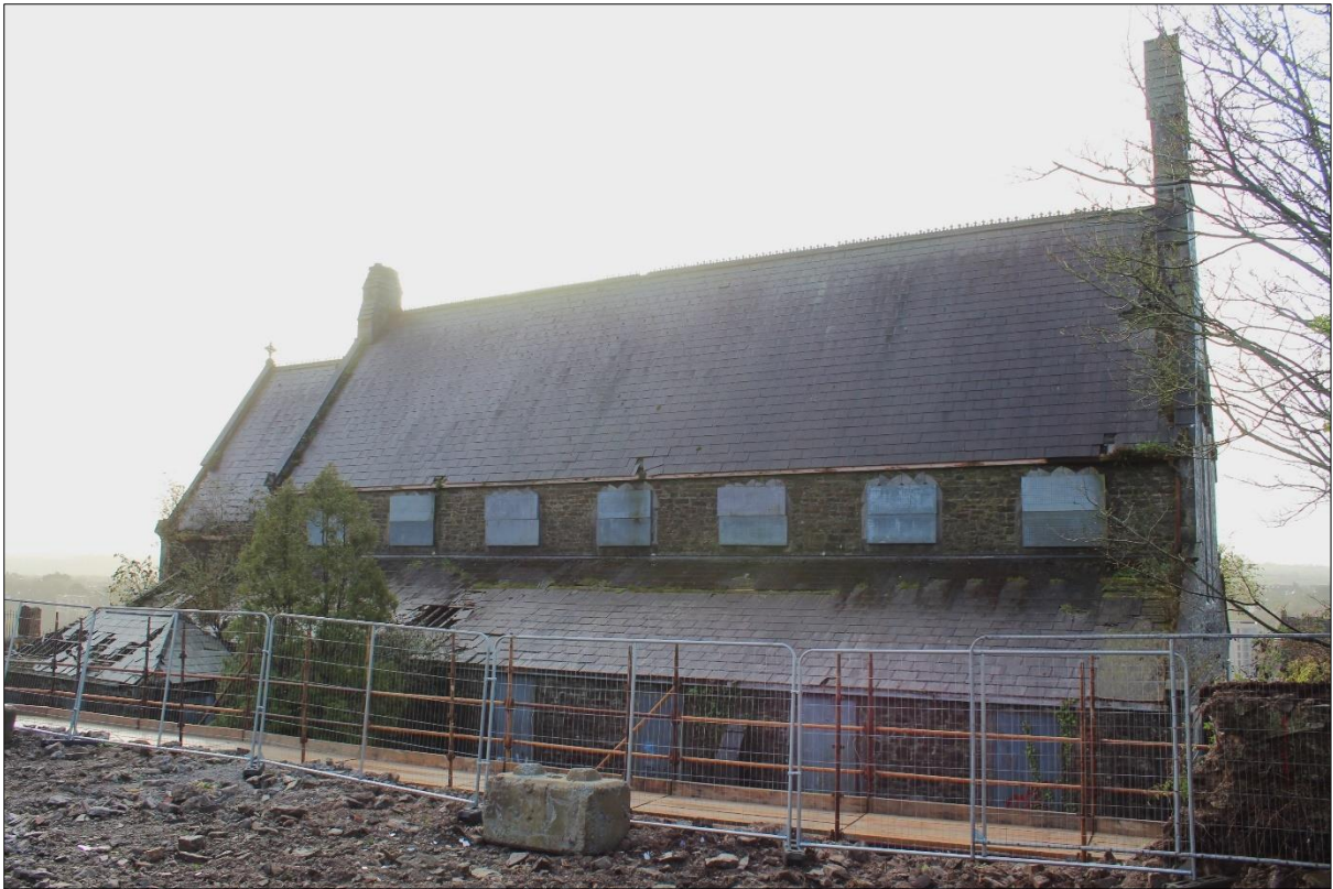
Plate 15: North elevation of former chapel
