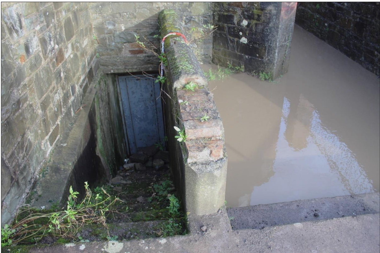
Plate 8: Steps down to basement level beneath east sanctuary
