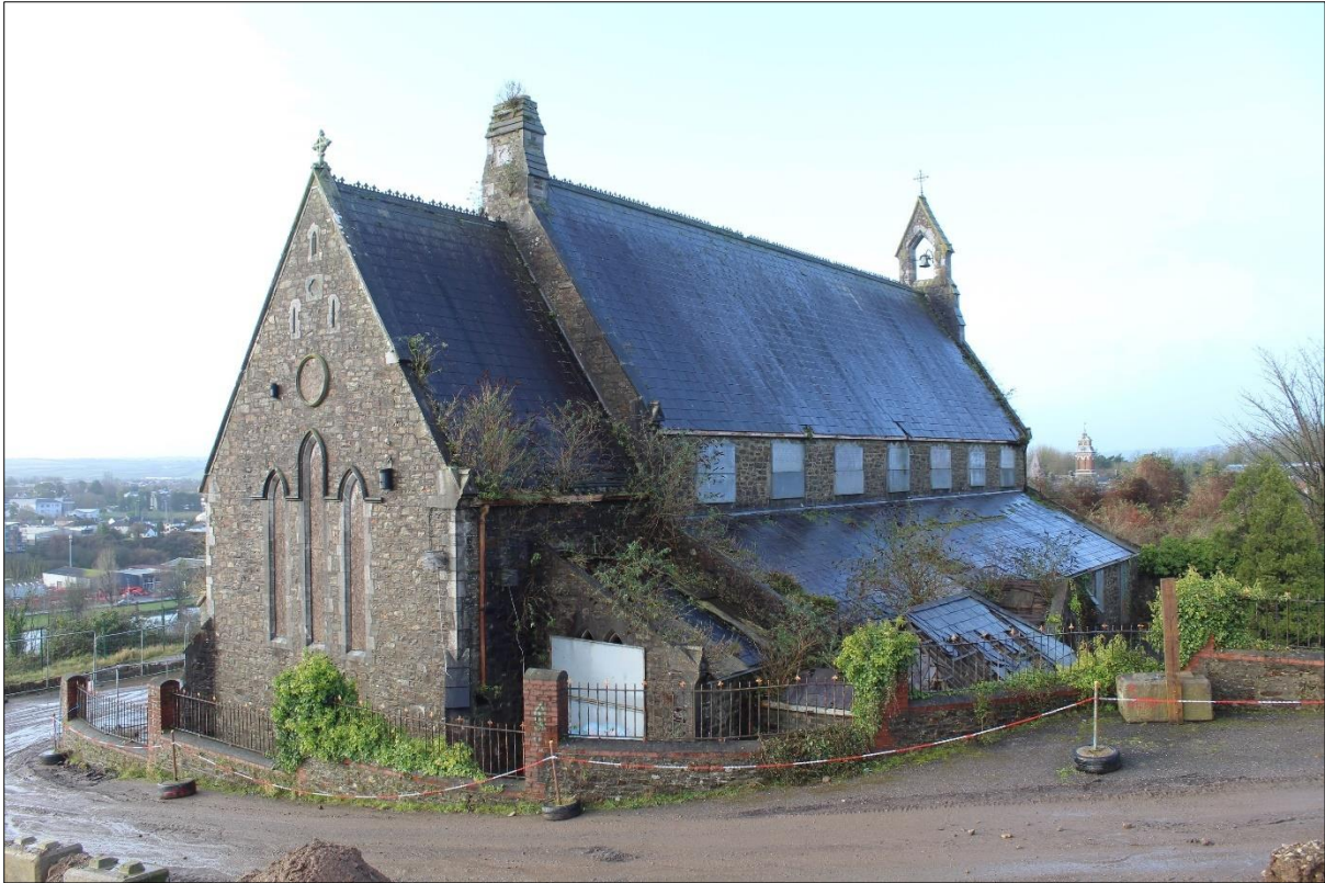
Plate 9: East gables and northern elevation of former chapel with curved brick and rubble masonry retaining wall supporting higher ground levels around the building with wrought-iron railings protecting the parapet.
