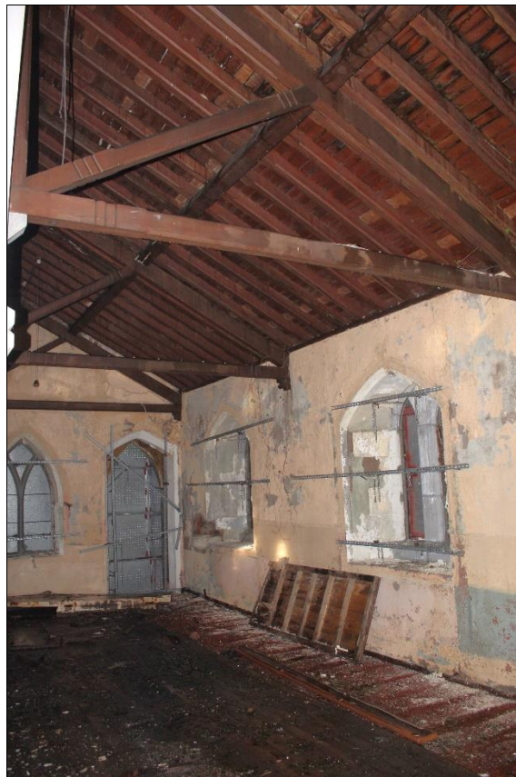
Plate 30: Western end of northern aisle
