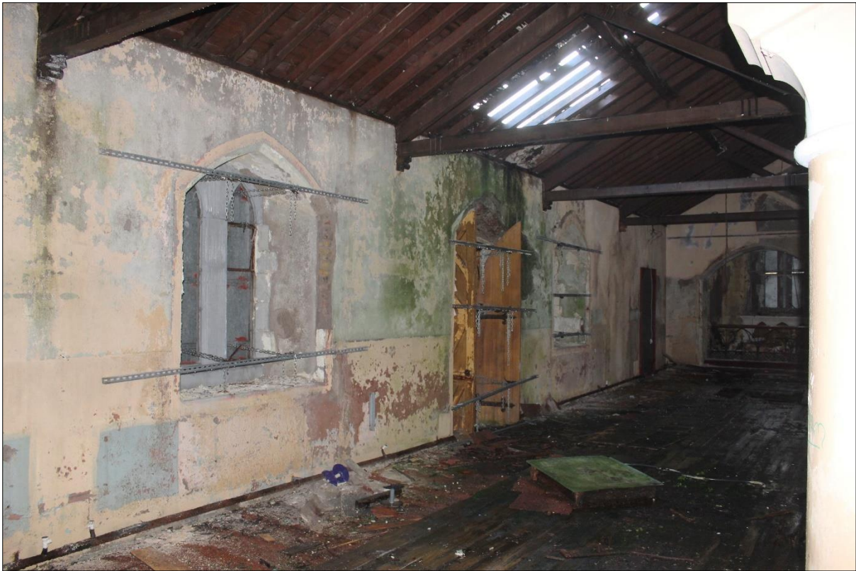
Plate 31: Rear entrance doorway off northern aisle.
