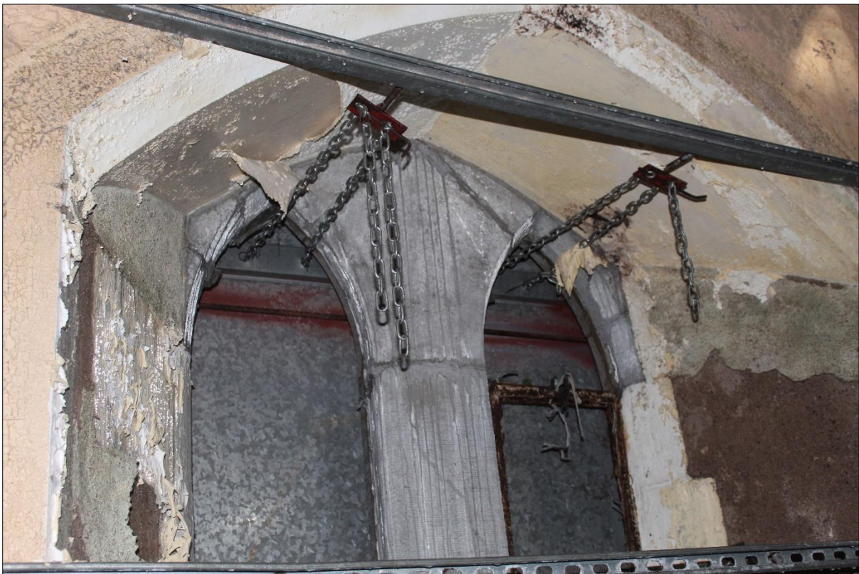
Plate 32: Detail of cut limestone frame to cast-iron windows on northern aisle
