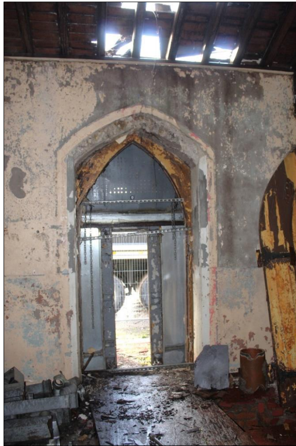
Plate 21: Doorway from southern entrance porch from within southern aisle.
